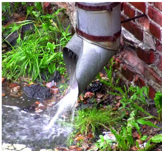
Fig. 6 The photograph on the left shows a problem downspout, and the drawing on the right illustrates a downspout that correctly drains water away from building foundations.
