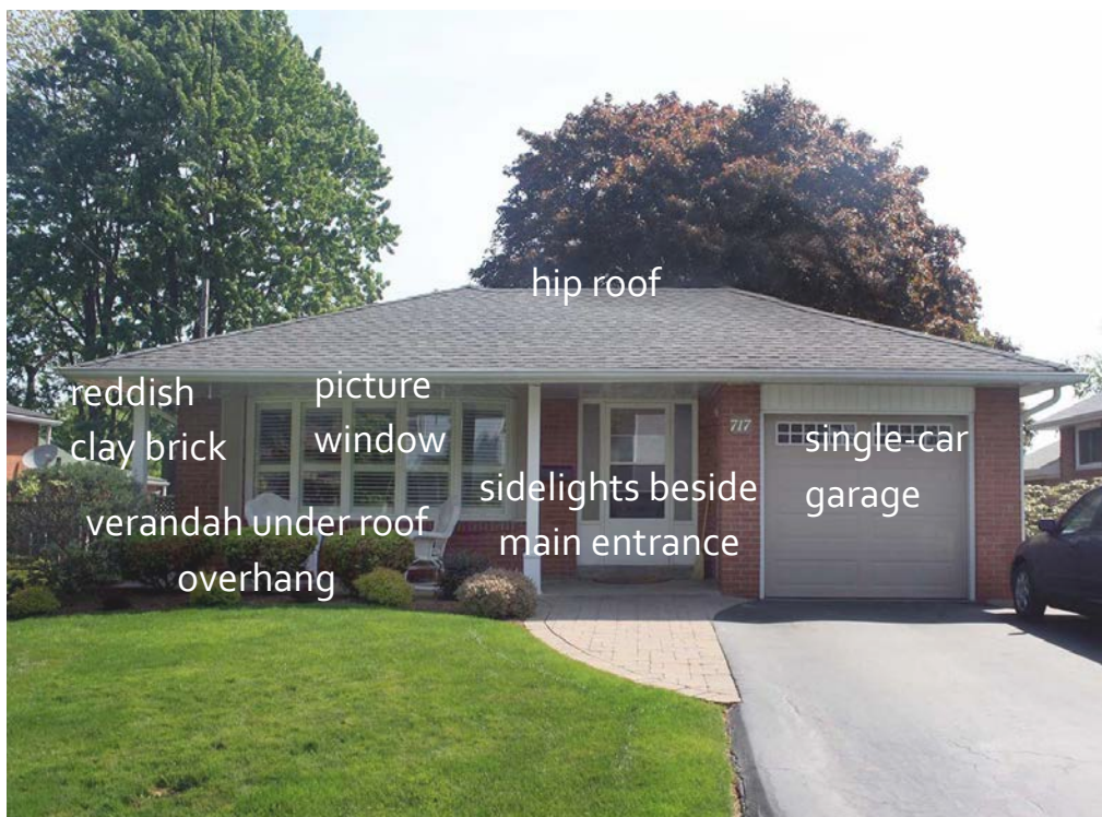
Fig. 5 A front facade view of a property classified as complementary (usual) is annotated with the house's features and wall cladding which are complementary to the neighbourhood's historic houses.
