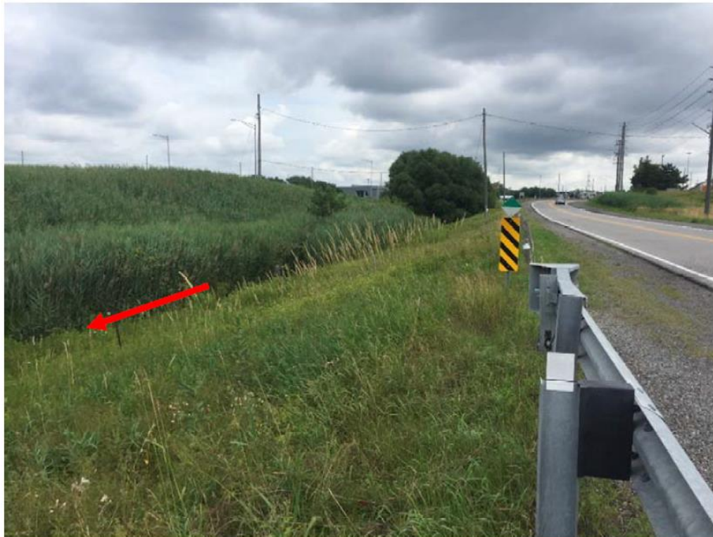
Figure 1-2 Road Embankment along Victoria Street
