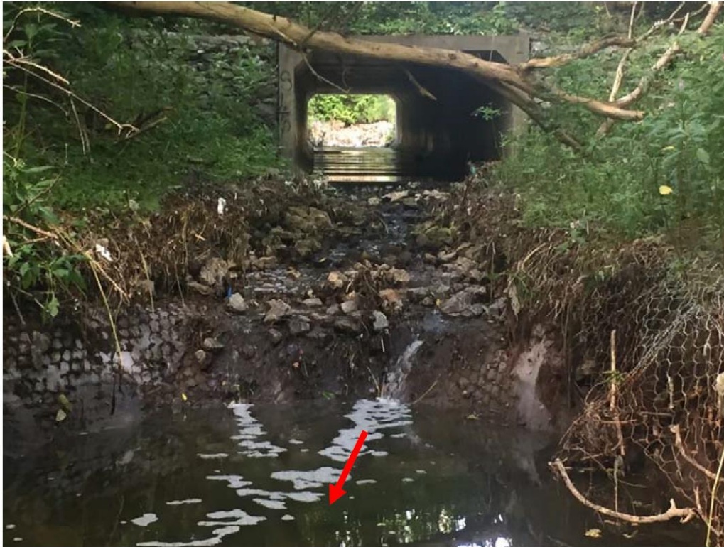
Figure 1-2 Channel Erosion at EB10
