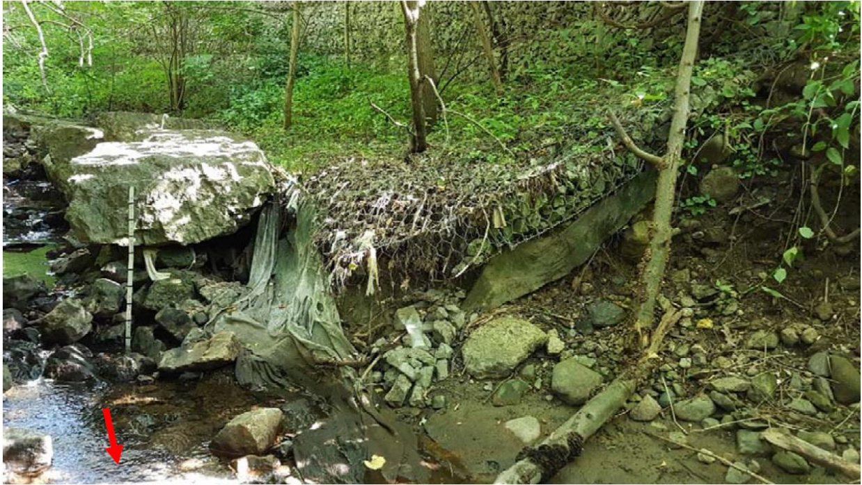
Figure 1-1 Armour Stone and Gabion Retaining Wall along Thickson Road
