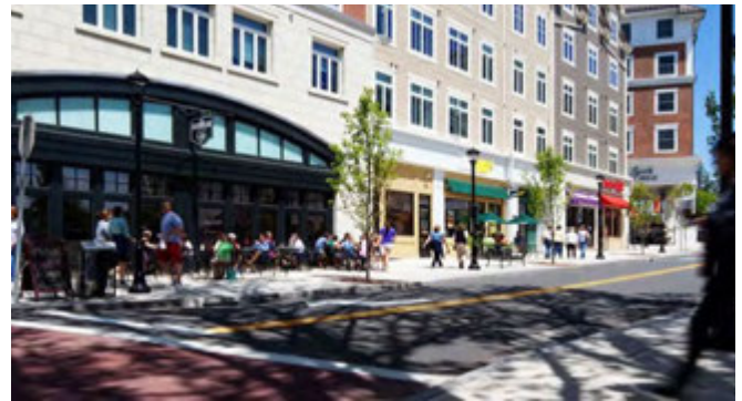
Precedent image of a mid-rise mixed use building along an enhanced pedestrian-oriented streetscape.
