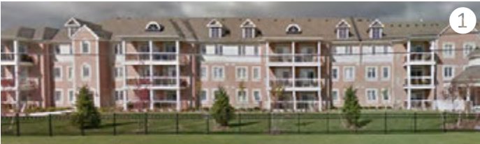
Existing medium density residential north of the site at Winchester Road West.
